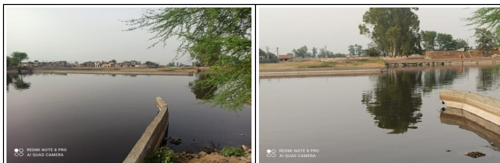
Storage and Sedimentation tank filled up with waste water of pond (16 March 2021)
